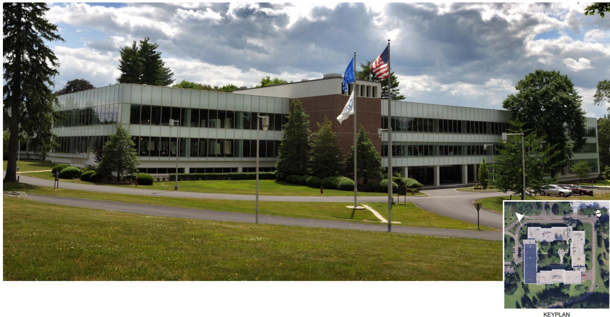
View of the main building looking south west
