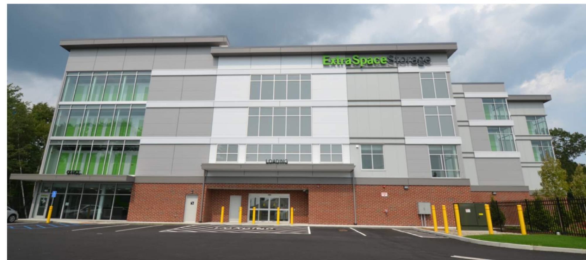
GLAZING SYSTEMS TYPE: CLEAR AND SPANDREL
