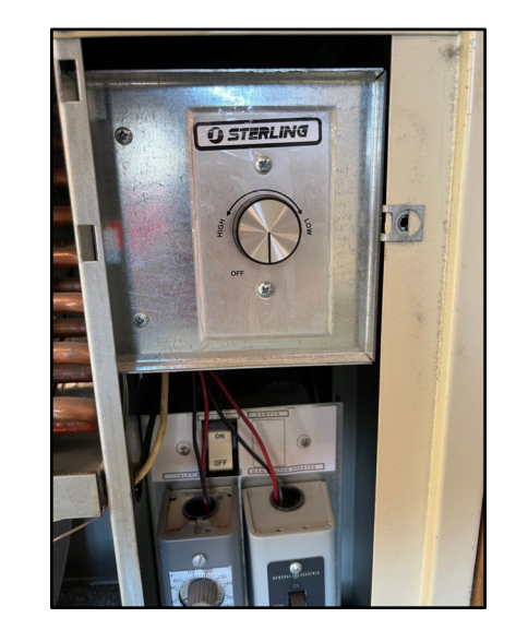
9 TYPICAL CABINET UNIT HEATER CONTROLS M-701 NTS
