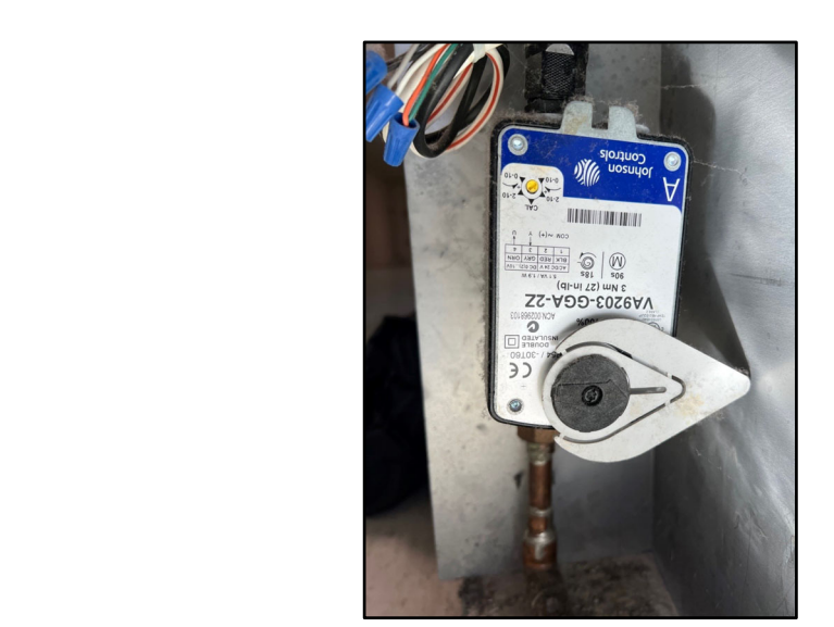
4 TYPICAL VALVE OPERATOR M-701 NTS
