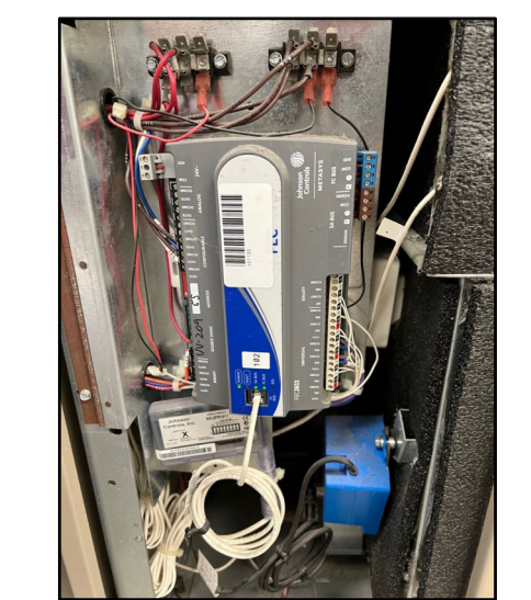
2 TYPICAL UNIT VENTILATOR CONTROLLER M-701 NTS
